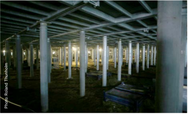
◀ The surface for the equestrian Olympics arena at Greenwich, London in 2012 was developed with the aid of mechanical surface testing described in this guide, and conducted by scientist members of the reference and review groups listed on page 4 and 5. A unique feature of this surface was the fact that it was not laid on the ground but on a platform (see inset) above it. This also posed a main challenge regarding the arena properties.
